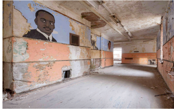
Photo credit: Noah Vaughn Jacob Riis Elementary School, Chicago. Demolished.
