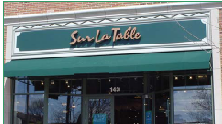
Contrasting, non-illuminated pin letters maintain the character of the existing storefront façade (2c)
